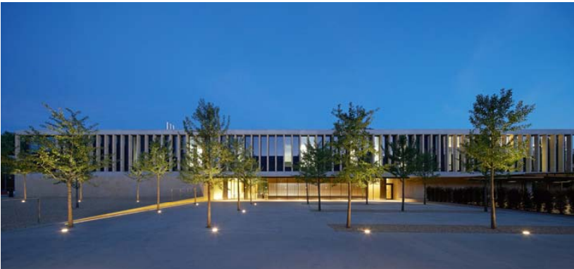
Image 5 – The Sainsbury Laboratory, Cambridge, UK, in its new monastic serenity (reproduced from: http://www.stantonwilliams.com/data/projects/372/img2.jpg ).
